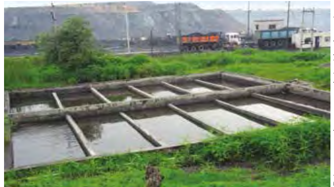
Primary settlement tank inside the mine
