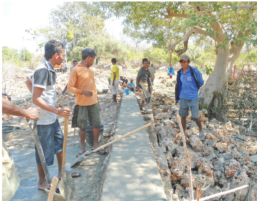
ROAD CONSTRUCTION IN SEMAU ISLAND.
