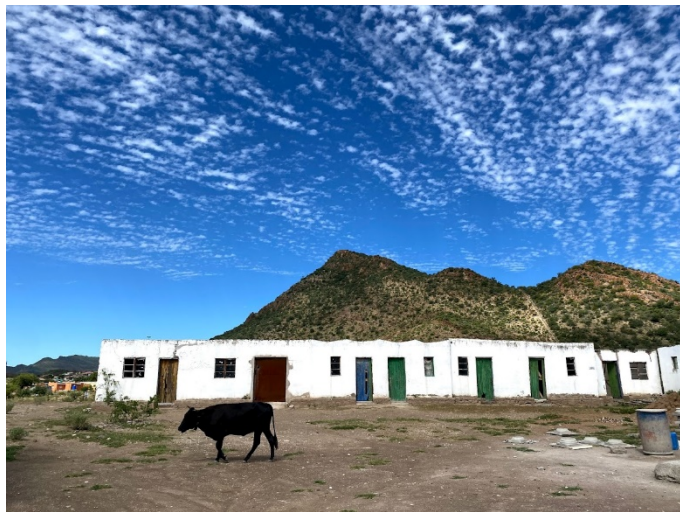
Figure 5: Abandoned rental units near Bokoni Mine, Limpopo
